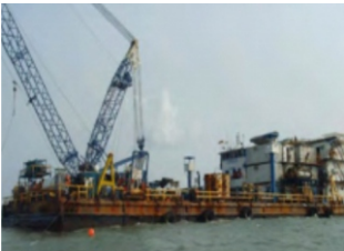
Enikkom Construction Limited MV Donaux offshore work Barge.
